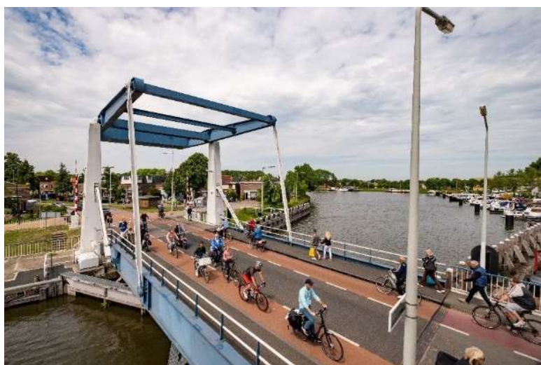
Figure 1. A movable bridge in the Netherlands (Copyright: Michiel Wijnbergh).
